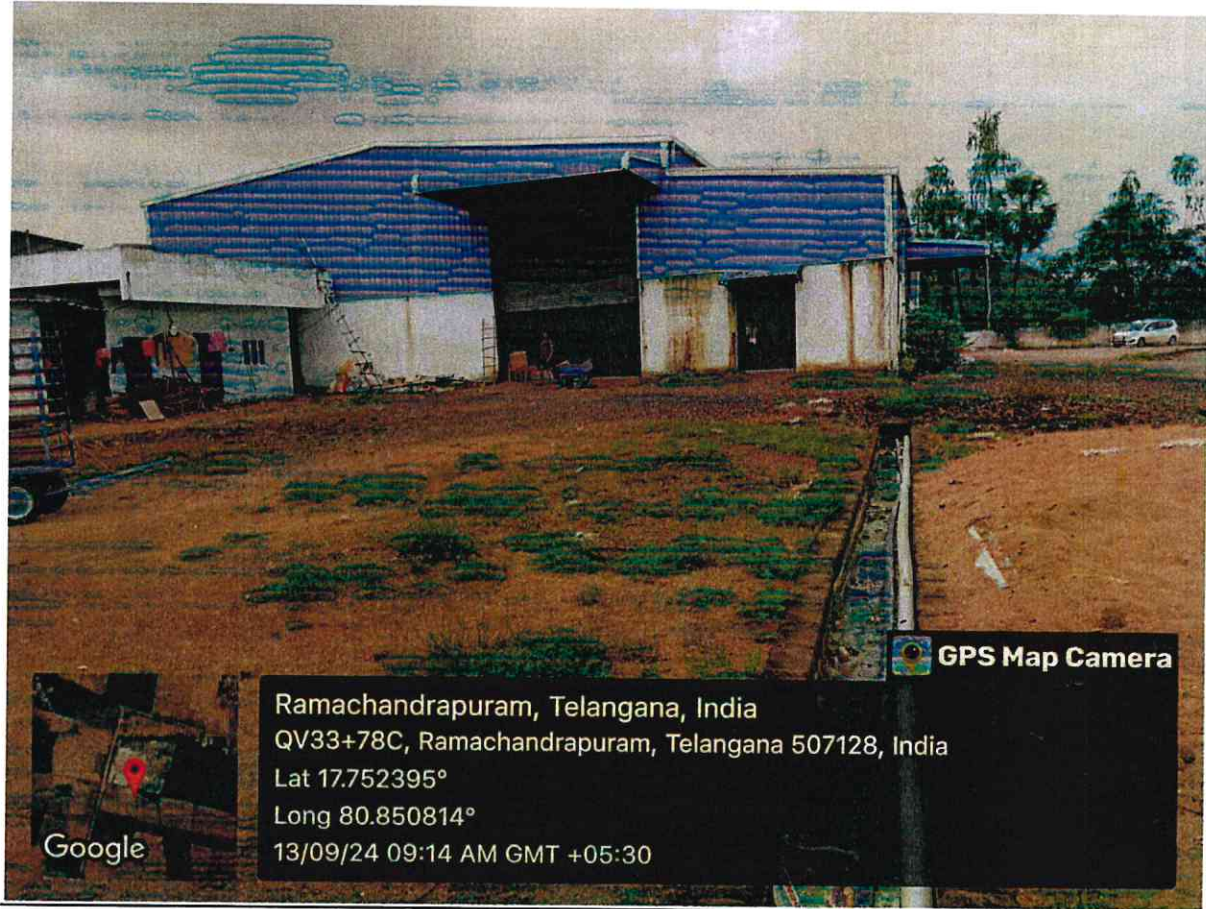
Washings drained water routed to settling tank
